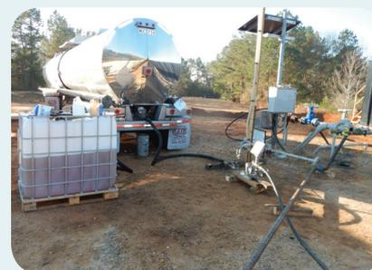
Formulation truck directly connected to injection pump for in-line mixing and direct injection of the foaming formulation.
